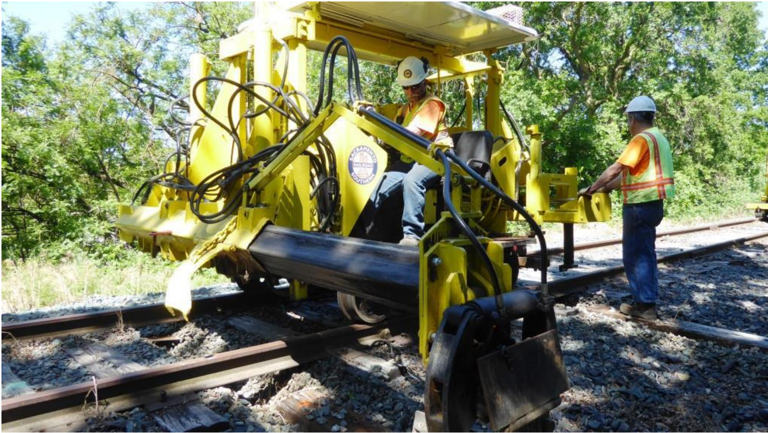
The Jackson 125, under Joe's expert touch, pulls old rotten ties from under the Sutterville Line
