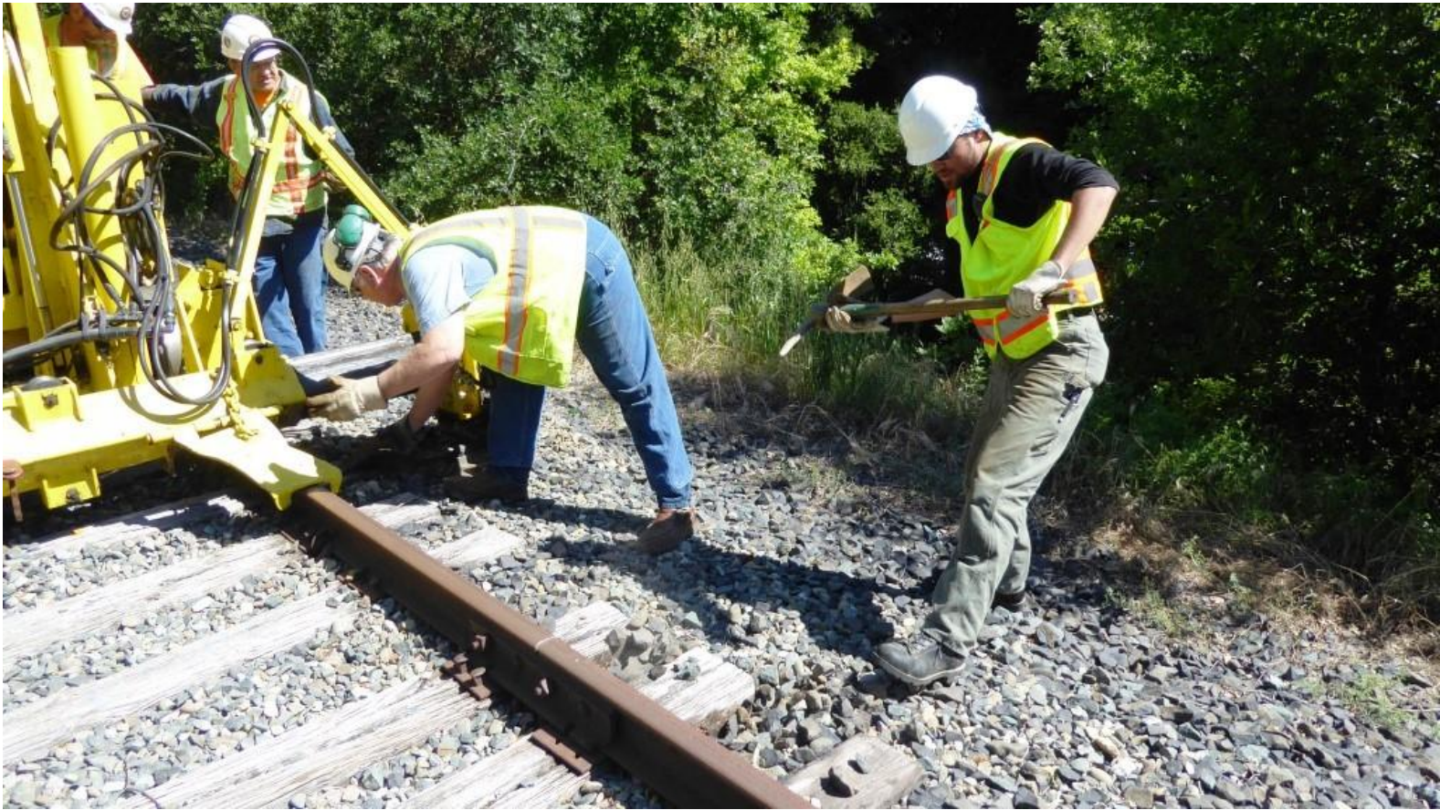
Kyle digs out the tie-ends to make it easier for the 125 to grab them
