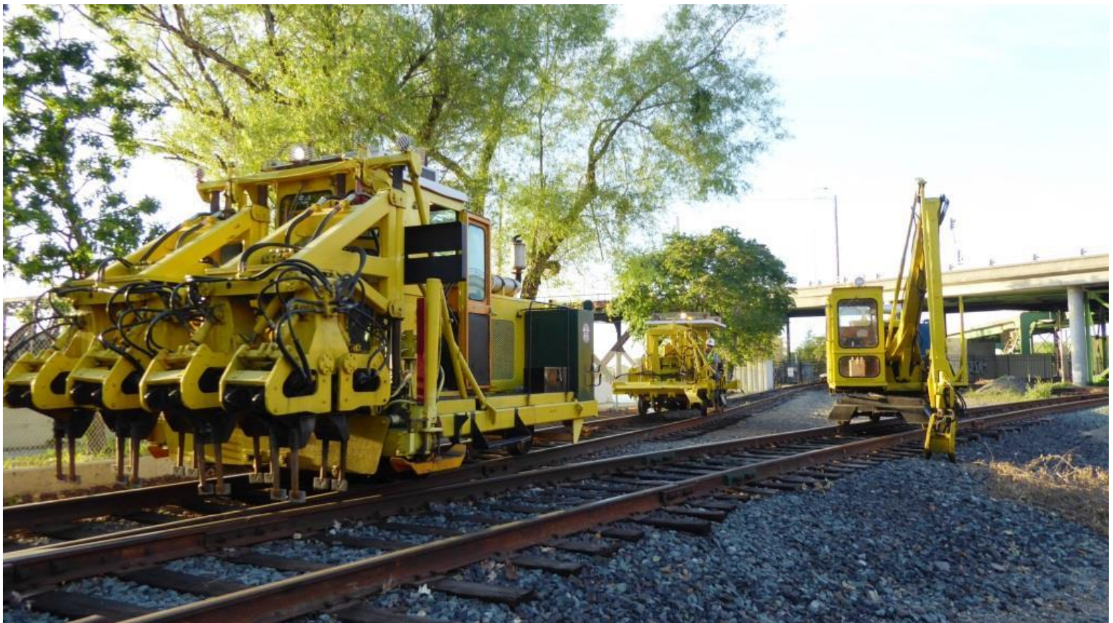
Mike H. get the tamper moving so that Joe can bring the 125 down the hill
