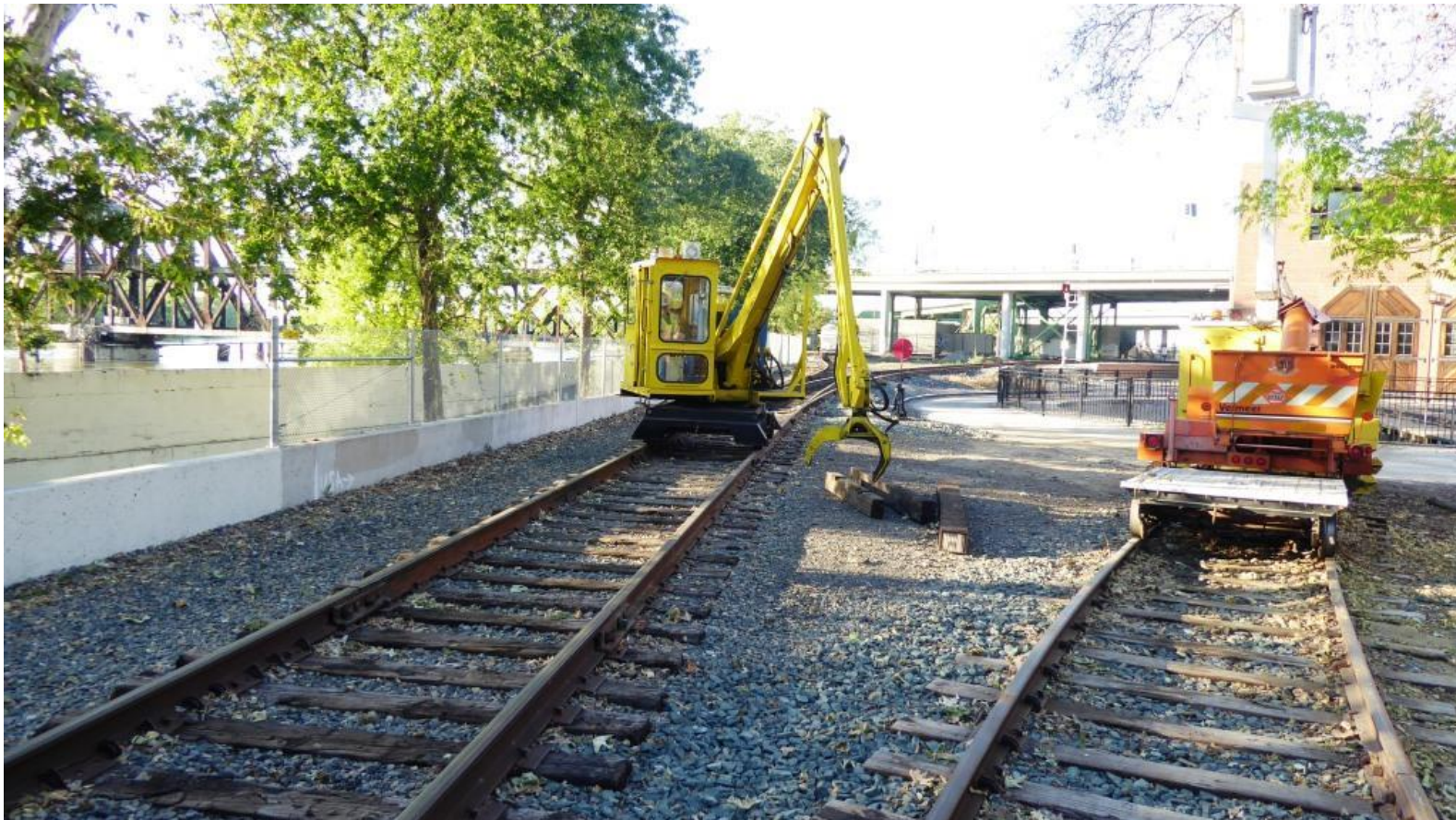
For the big equipment shuffle, Mike H. brings the tie-crane down the hill
