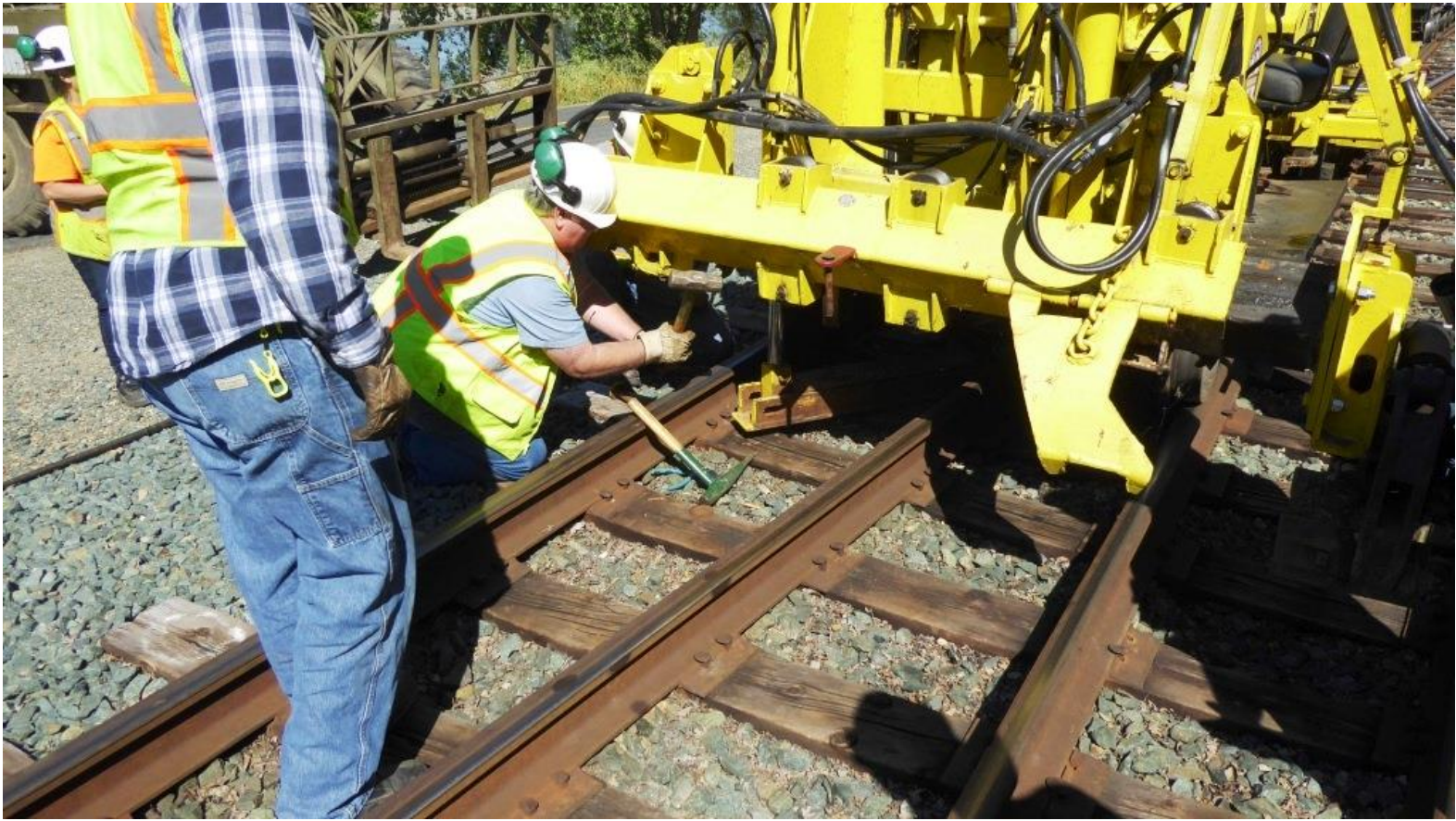
The lift-cylinder and ram on the 125 would not retract, so, Chris works to remove it so that the Team can move on
