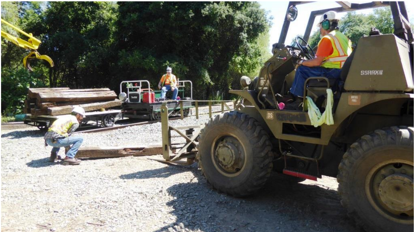
At Setzer, Matt B. lifts the end of a dead-tie so that Ed on GM2 can get the forks under it
